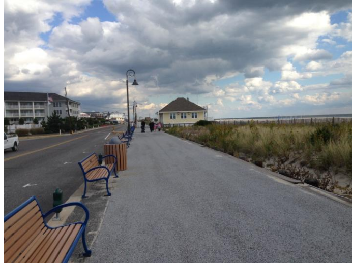
Figure 25 - Asphalt Bicycle/Pedestrian Path at the Beach Promenade
