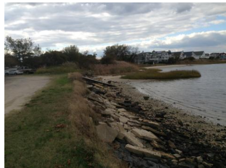
Figure 6 - Cape May Harbor
