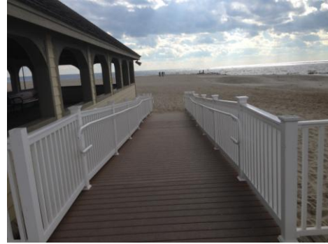
Figure 2 - Accessible Access at Beach Pavilion
